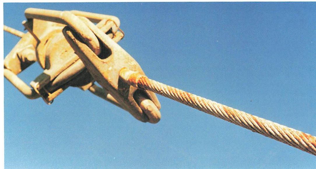
Guy rope and insulator assembly corrosion 7NT Kelso.
