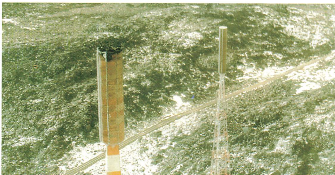
Lightning damage to ABNT3 Mt. Barrow radome. Commercial antenna TNT9 (R) escaped damage.
