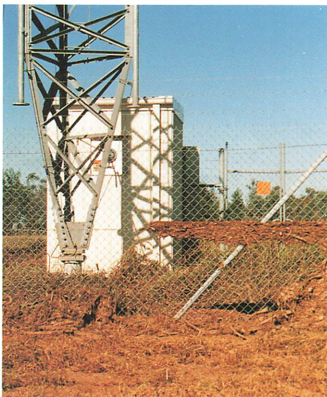
Debris indicating level of flood waters at 4CH mast base.
