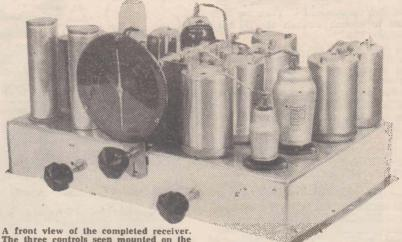
A front view of the completed receiver. The three controls seen mounted on the side of the chassis are (from left to right) the tone control, the main tuning control and the volume control.
