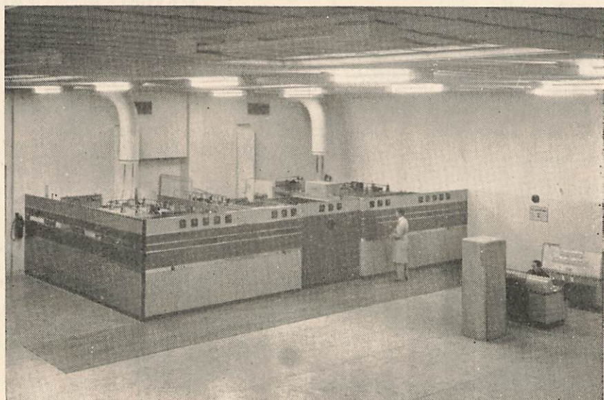
This view depicts the 50 kilowatt Radio Australia transmitter, VLC.
