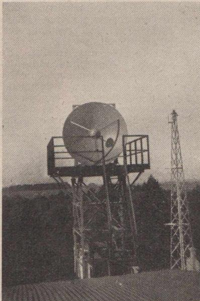
Micro-wave Parabolic antenna system as used for television relay links.
