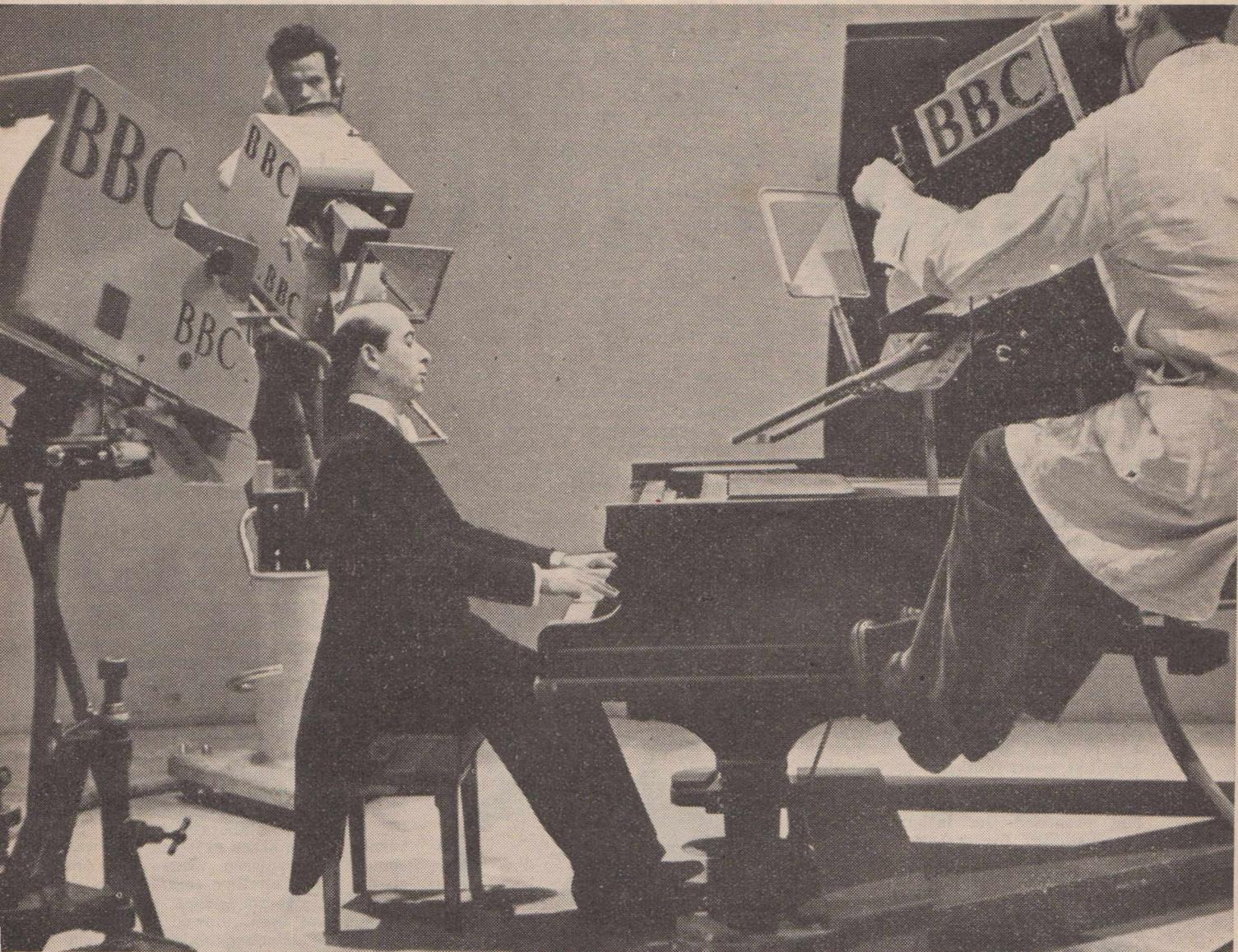
★ B.B.C. Television Service. The well-known pianist Monia Luter before the cameras at Alexandra Place, London. The mask frames seen in front of two of the cameras are used when special effects are required for different parts of the televised picture (e.g. "vignetting"). —Photo by courtesy of the B.B.C.
