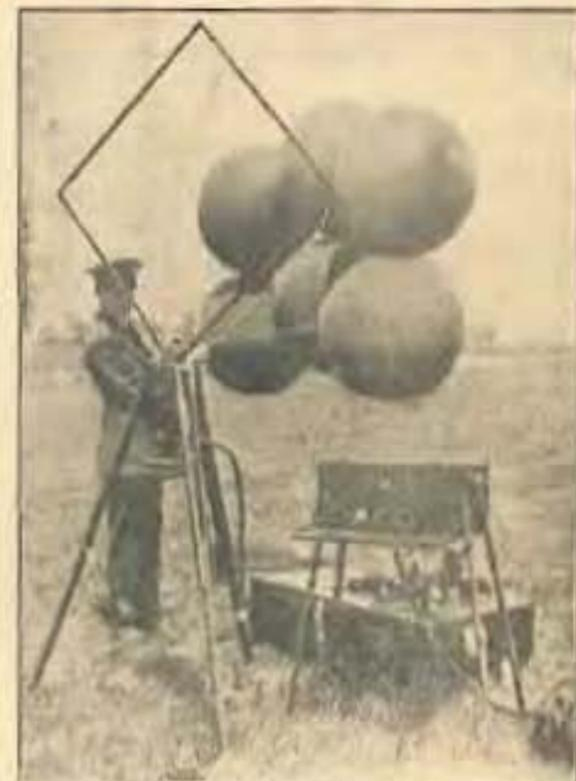
The complete apparatus, showing the direction finder loop, the receiver, and the miniature transmitter attached to the balloons.
