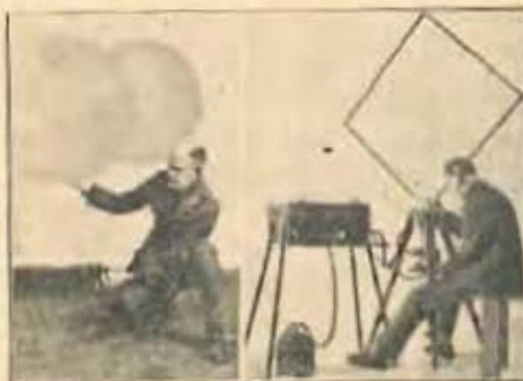
On the left—An Officer sending up the balloons with the transmitter, which weighs only one pound. At the right the ground apparatus can be seen ready for operation.
