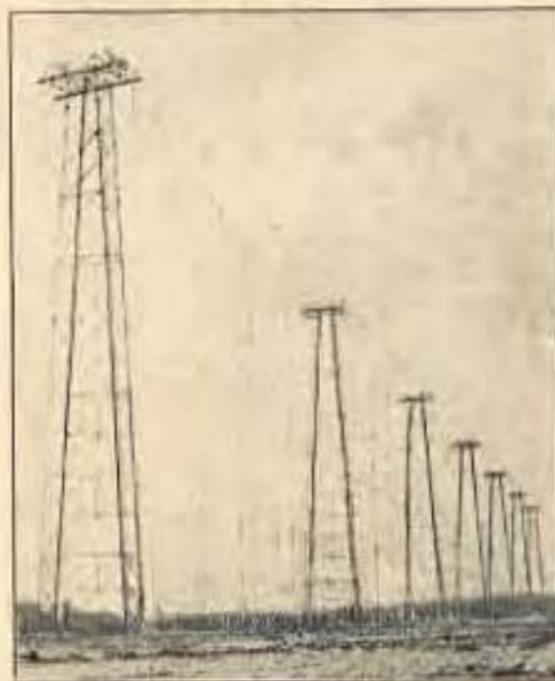
Europe, and others of seven similar masts serve South America and other continents. 10,000 volts are used on the plates of the transmitting valves. In the illustration here are shown the seven 180-foot masts with mesh aerial that was used to communicate with Sydney recently.
