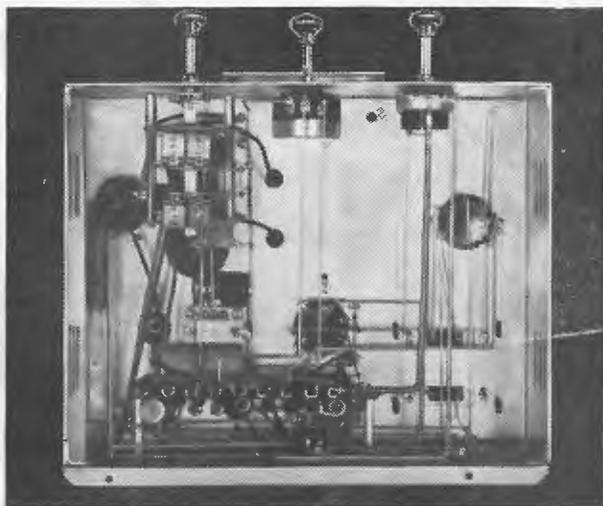
Above: An under-chassis view of the completed kit, showing the simplicity of the assembly and wiring.
