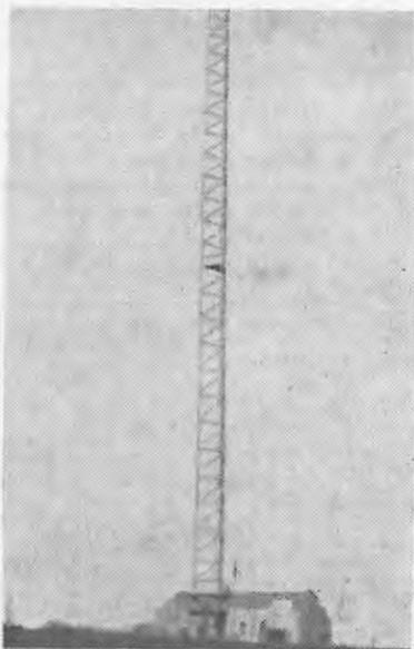
This aerial mast belongs to 1YA, Auckland, which operates on 650 k.c. with a power of 10 k.w.
