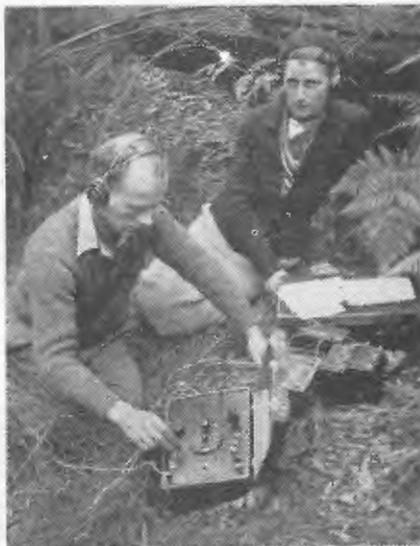
This photo shows Geo. Choules (2BH) operating the crystal-controlled transmitter designed by him for portable operation.
