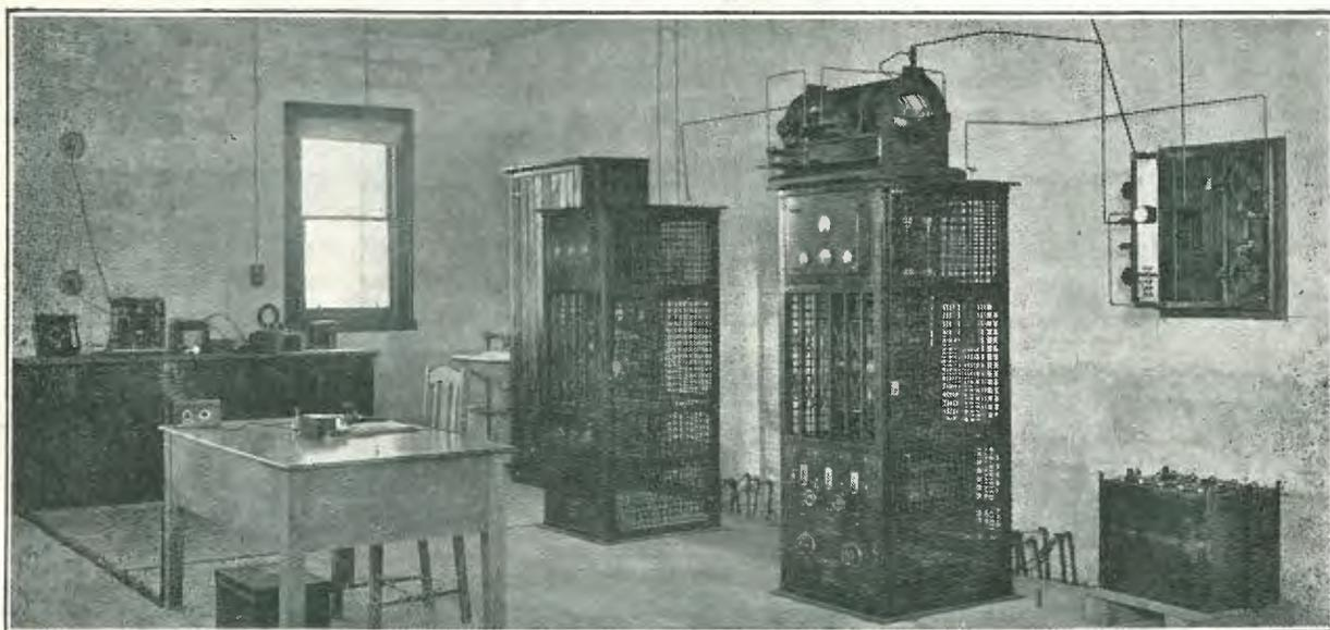
A corner of the station's operating room. On the right is the  $\frac{1}{2}$ Kw. Oscillator Panel, while further back is the Modulator Panel.
