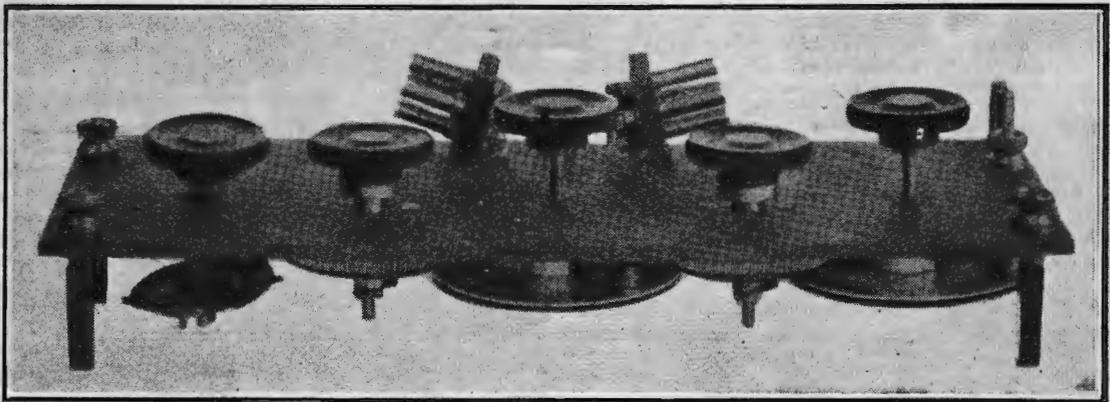
Complete two-valve receiver of particularly simple construction.
