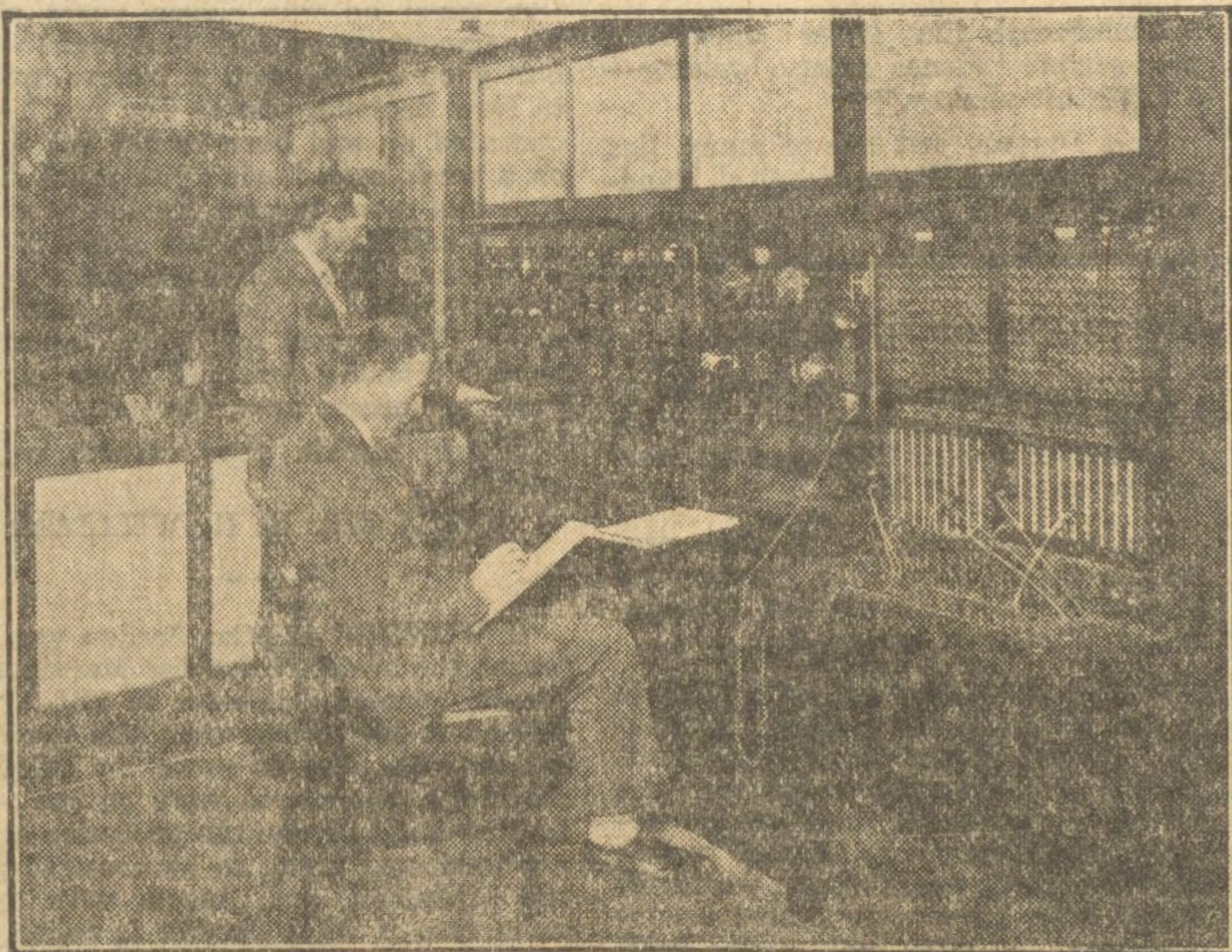
The control room at 2FC, showing the unique and vastly intricate panel system. From this panel is controlled all the various outside relays, including country programmes, land recitals, theatres, etc. Individual control of each of the half-dozen microphones in the three studios is also possible from this panel. The chief engineer, Mr. Burbury, is seen standing.
