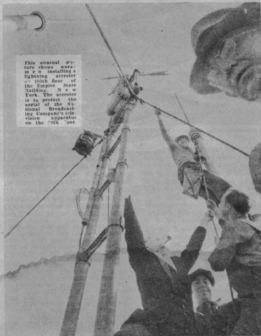
This unusual picture shows workmen installing a lightning arrester on the 105th floor of the Empire State Building, New York. The arrester is to protect the aerial of the National Broadcasting Company's television apparatus on the 66th floor.
