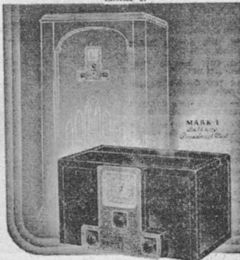
**MULLARD** Master Unit Mark 1 is a high-grade 7-valve battery-operated broadcast receiver of unique construction and performance. Valves are part of the unit, but accessories, such as batteries, cabinet, speaker, are not supplied, and are left to individual choice according to requirements or circumstances.
