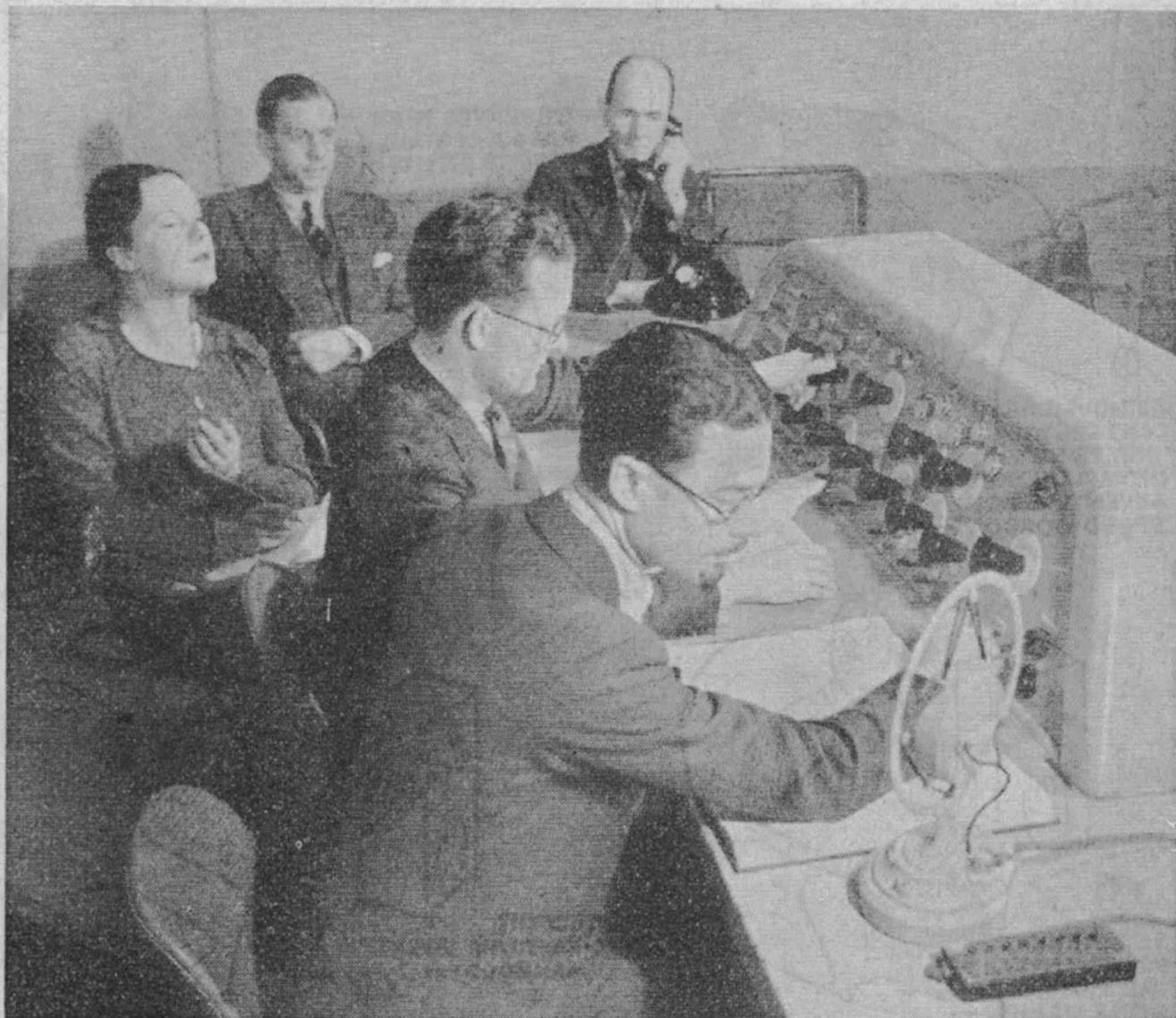
In the dramatic control room at the B.B.C., London, Val Gielgud, the producer, is at the microphone with the script before him, operating the mixing panel which brings in the effects from the effects studio and the actors' voices from another studio. He is assisted by another operator, a time-keeper with a stop-watch, the author (perhaps), and a monitor.
