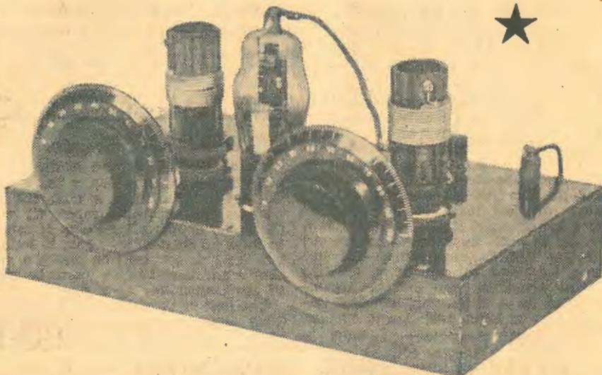
*The buffer stage. The grid coil is at the left and the plate coil at the right. Filament and high tension connections are made to terminals at the rear.*
