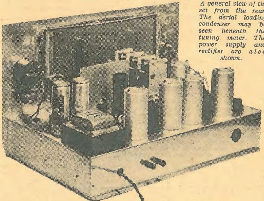
A general view of the set from the rear. The aerial loading condenser may be seen beneath the tuning meter. The power supply and rectifier are also shown.
