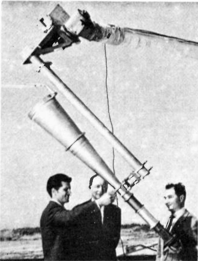
Close-up of horn antennas of Intelsat IV.
