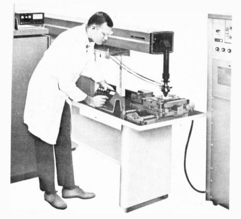
Fig. 4. 250W CO2 laser cutting unit.
