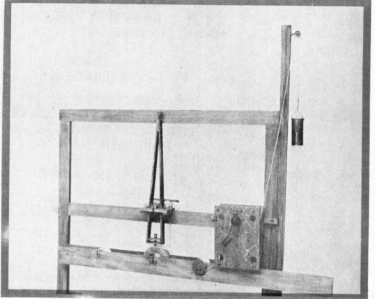
Fig. 1. The receiving terminal of Morse's first telegraph. The falling weight drives the paper strip past the triangular shaped pencil holder. Current received by the coils halfway up this holder cause the beam to deflect making a mark on the trace.
