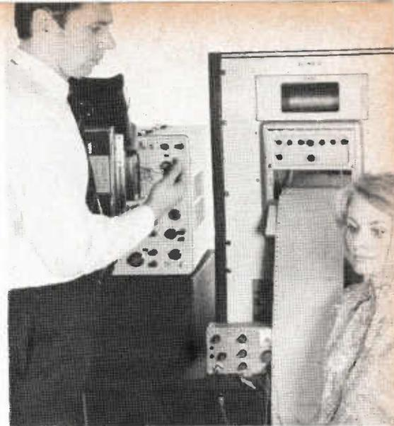
Fig. 9(a). Layout of apparatus for recording the electroretinogram and the visually evoked cortical potential. (Illustration after Millodot).
