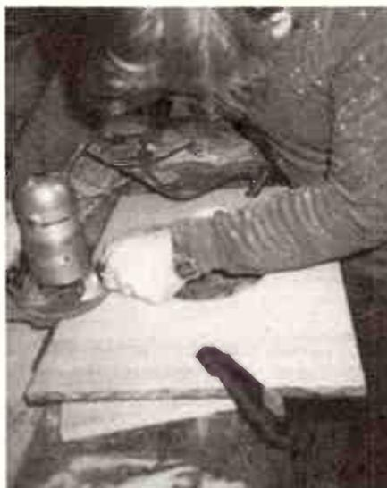
*Routing the sides of the front panel to obtain a flush fit.*
