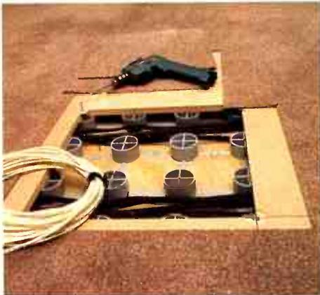
CoDesign offers two advanced and flexible access flooring systems to handle the cable management requirements of the automated office of today and tomorrow.
