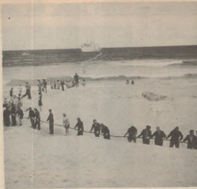
Far left, the Cooke and Wheatstone telegraph instrument as used on the London railway, 1845. At left, bringing the Australian end of the Trans-Tasman cable ashore, Bondi Beach, 1975.
