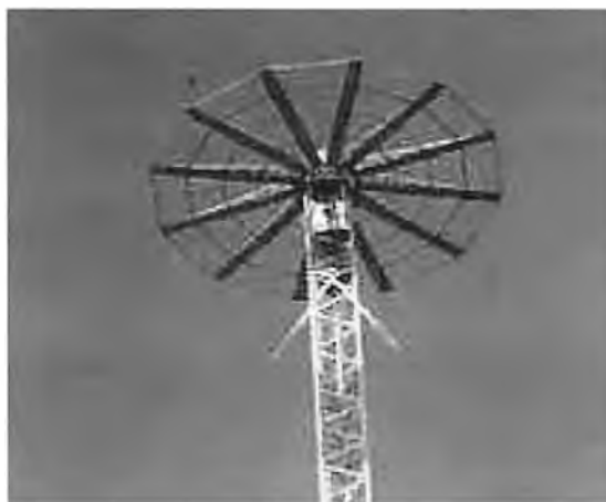
A typical broadcast vertical capacitance hat.
