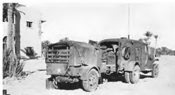
A Chevrolet panel van with SCR-299 and 'Ben-Hur' trailer containing a petrol driven generator photographed in North Africa in 1942.
