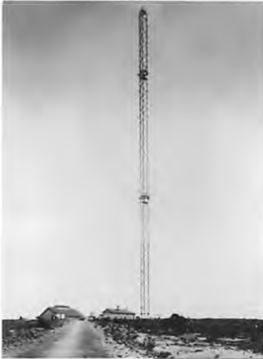
The 120 m tall, steel, guyed aerial mast at Wireless Hill, circa 1912.
