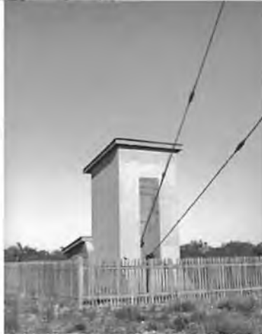
One of three 200 ton concrete guying anchor blocks for the steel mast, circa 1912
