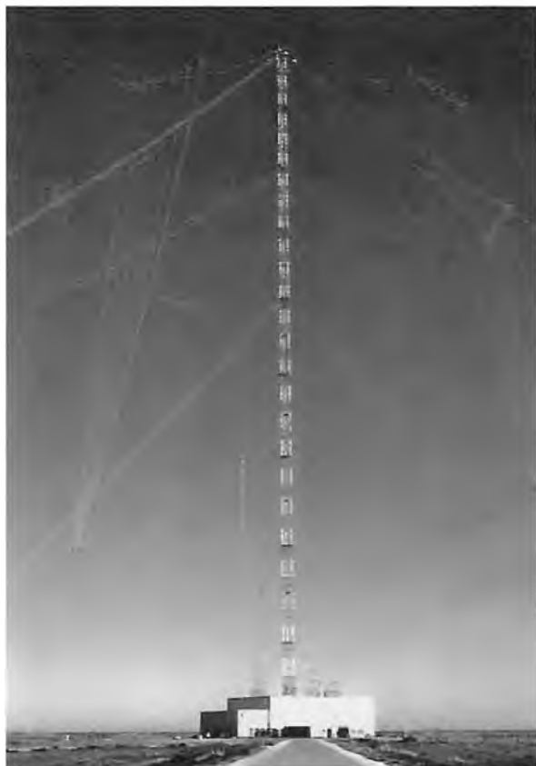
Tower Zero of the Trideco VLF antenna system which consists of 12 towers grouped around this 13 th central tower. Each of the towers is 304 m in height.
