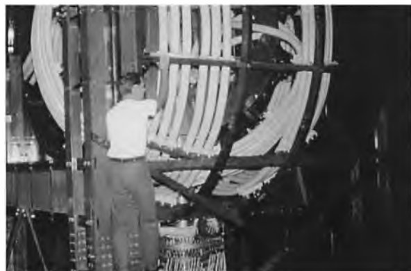
A US sailor climbing one of the variometers in a Helix house with Litz wire visible near his feet.
