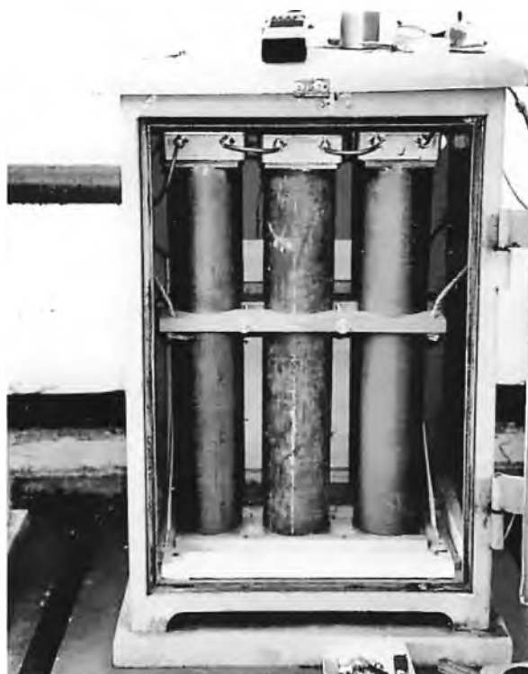
The duplexer cabinet and the six cavity duplexer.
