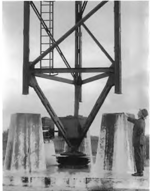
Photo of the concrete base of the original 120 m mast with sway insulator, taken in 1912.
