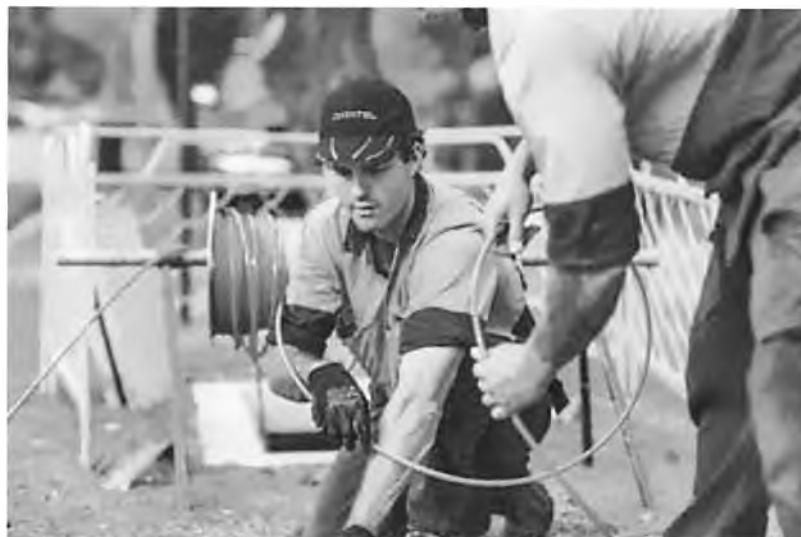
An NBN team installing fibre optic cable.
