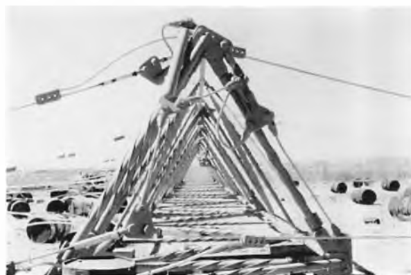
A VLF antenna system catenary, August 1978.
