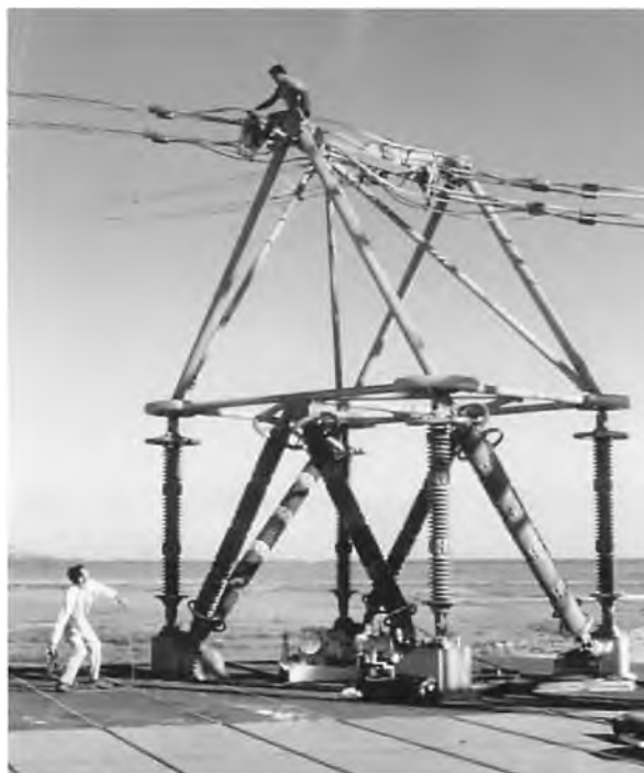
Antenna riggers working on part of the extensive VLF antenna system on the roof of the VLF building.
