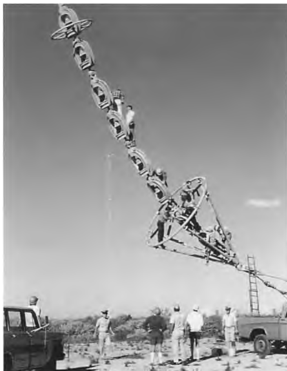
A maintenance crew working on insulators forming part of the VLF antenna system in 1972.
