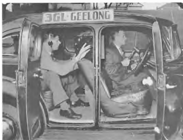
The car used in the 1948 broadcast of the Warrnambool Road Race, a 1939 Packard Model 1700 showing commentator Jack Dillon and 3GL chief engineer Jack Mathews adjusting the AWA FS 6 transmitter and receiver. 2
