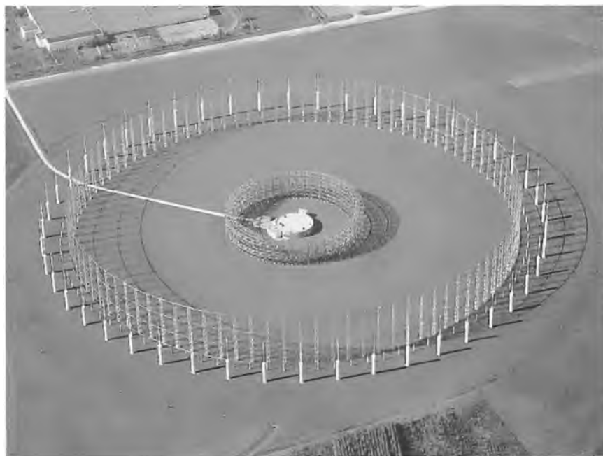
A typical Wullenweber CDAA antenna.
