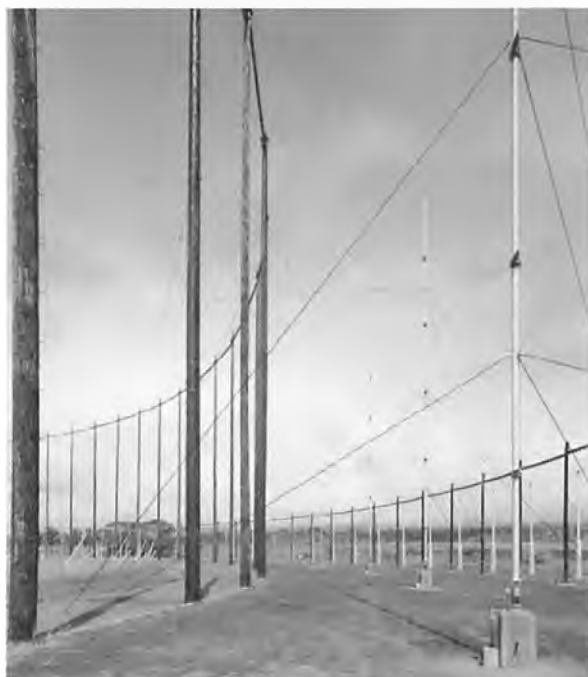
Detail of dipole antenna element (right) and 94 ft (28.7 m) low-band reflector screen poles (left); note the guy wires from the antenna element; viewed facing north northeast at the US Naval Base, Pearl Harbour, CDAA antenna system.
