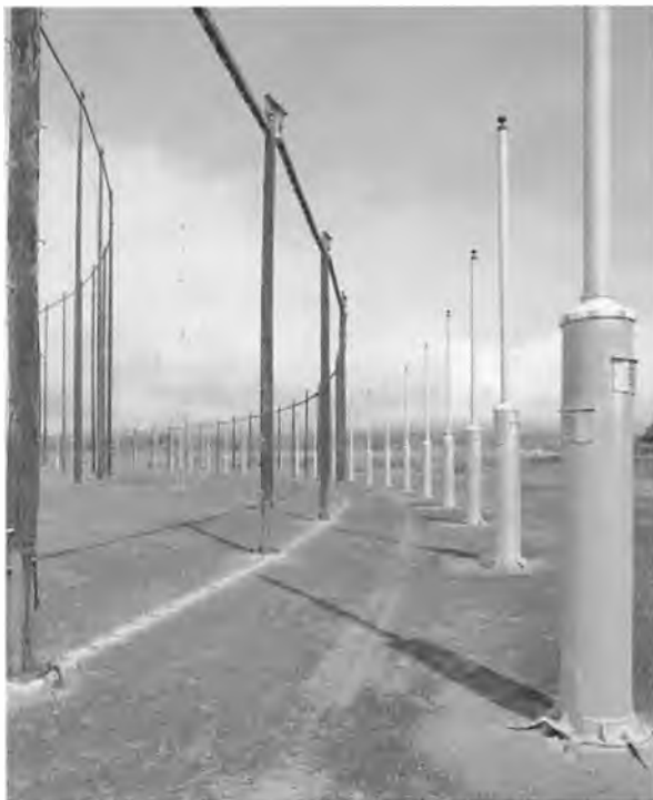
Detail of monopole antenna element (right) and 25 ft (7.6 m) high-band reflector screen poles (left), viewed facing northeast at the US Naval Base, Pearl Harbour, Naval Radio Station, AF-FRD-10 CDAA antenna system.
