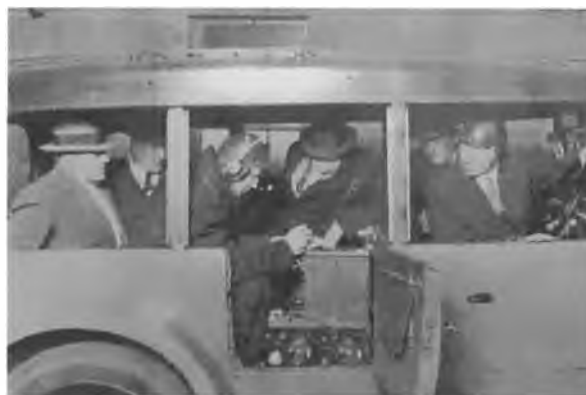
A close up view of a Daimler wireless patrol car with a full team of six officers on board. The trained wireless operator is taking down a message from a Morse transmission.
