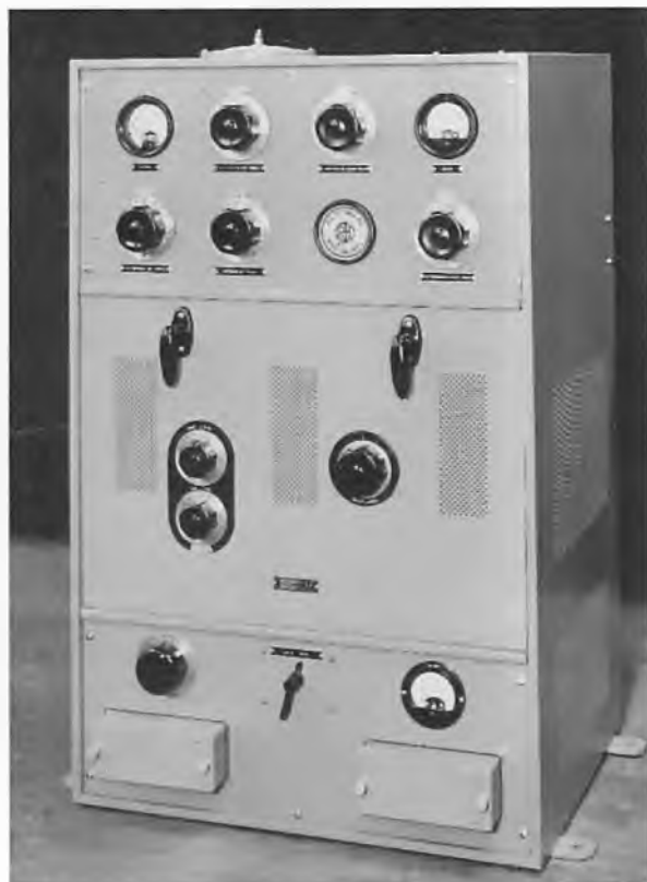
An NSF-Philips MZ33 HF valve transmitter made in 1939.
