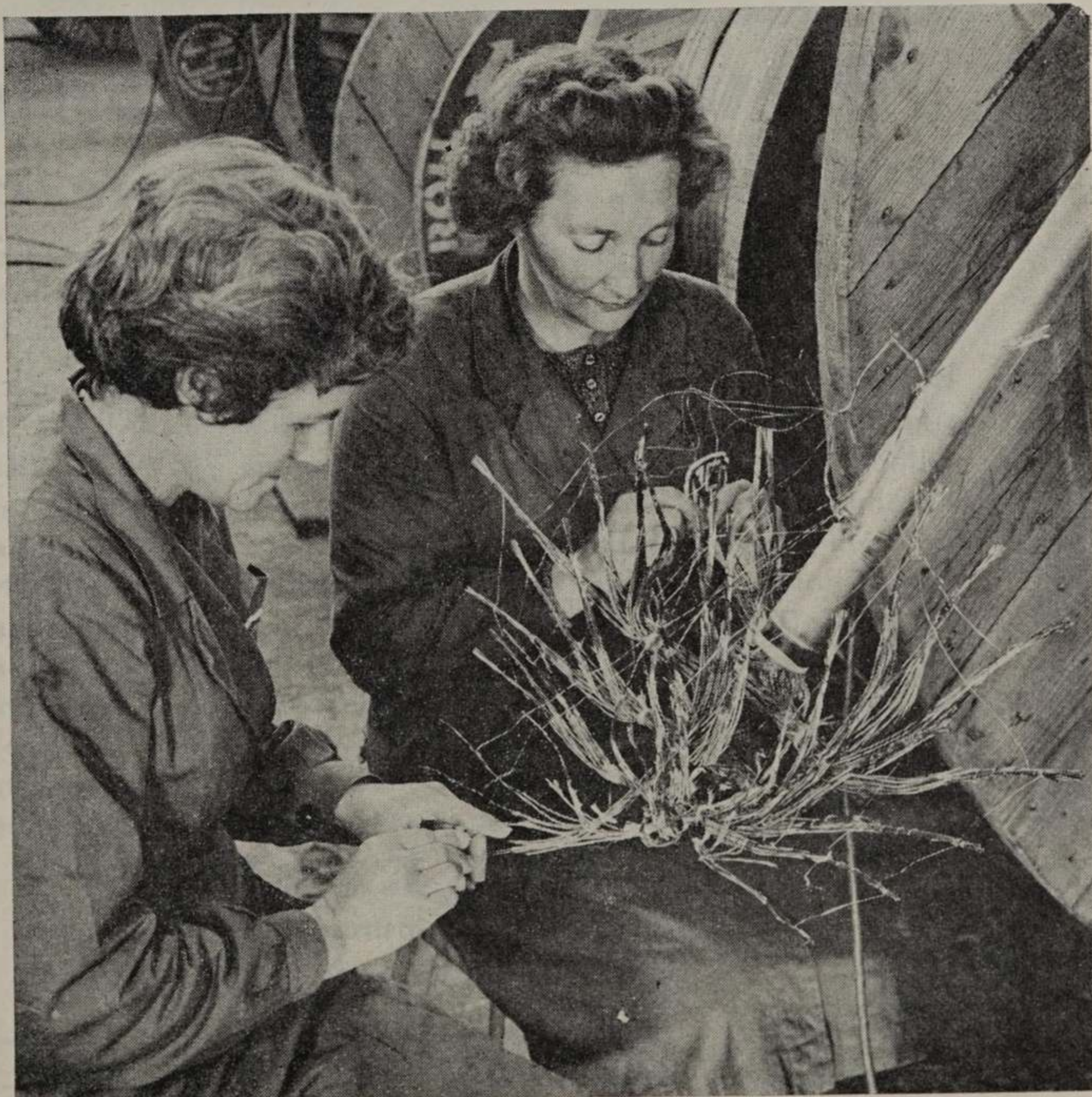
Below: A 300 pair 20 lb quad local type cable being prepared for 'final test'.
