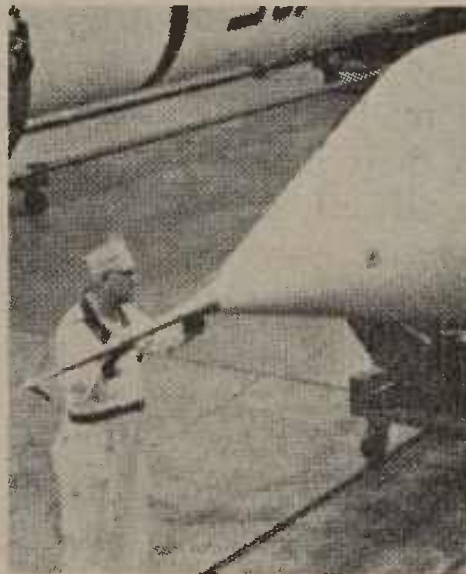
The transducer installed on a Redstone missile
