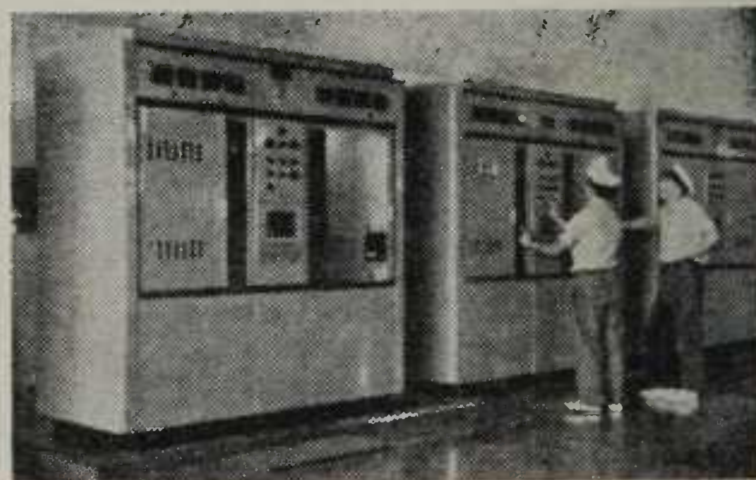
Royal New Zealand Navy personnel running up A.W.A. CTH7 5 KW Communication Transmitters after installation.
