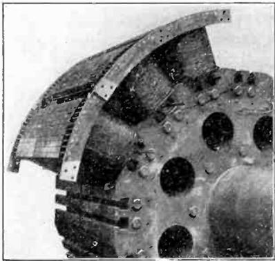
FIG. 13—ROTOR WITH LAMINATED SPIDER
