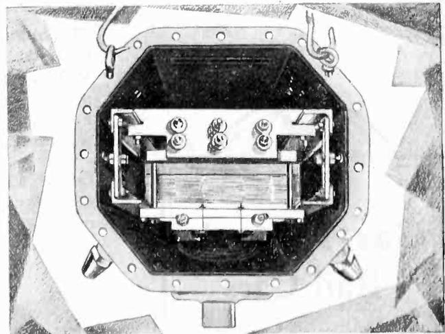
Wagner Subway-type Transformer, cover removed showing terminal board.
