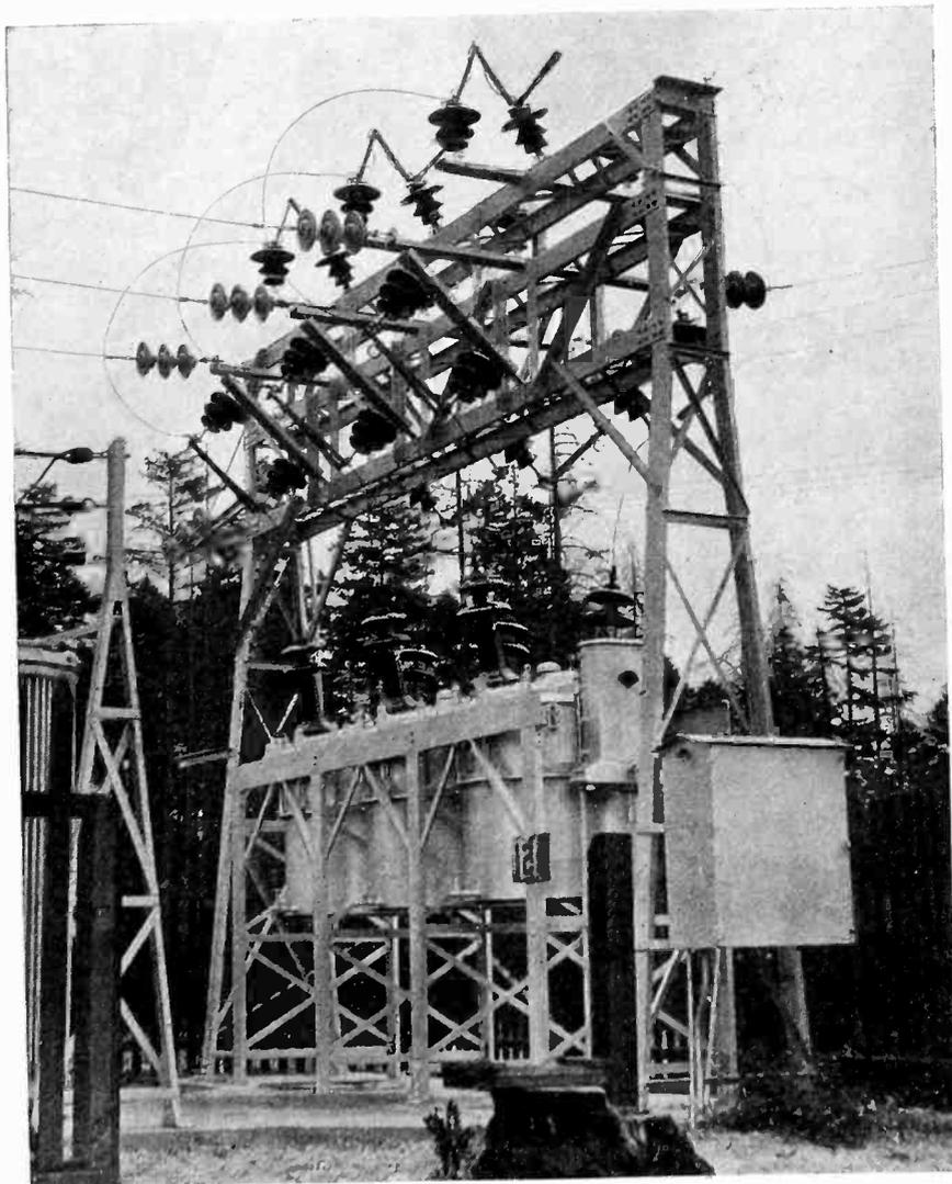
Pacific Type K By-pass and Type G Disconnects are shown on the structure.
