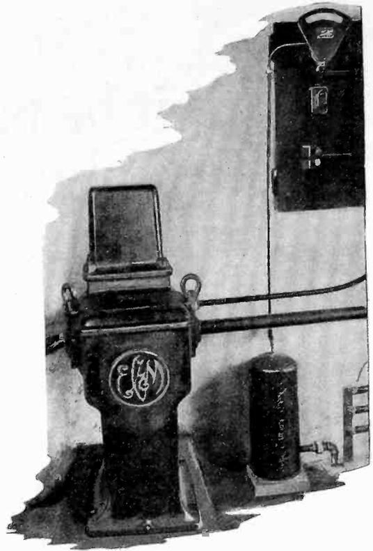
*Shown above is a typical EC&M Control installation for a village water system. The Altitude Regulator starts and stops a pump through the EC&M Automatic Compensator.*
