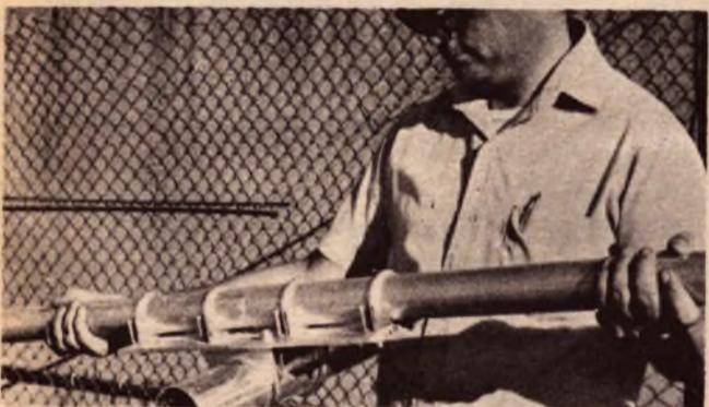
Our 40 meter element to boom clamps are constructed of aluminum bar plate 1/4" thick, 5" by 18" long. The element is secured with 6 ft. coupler and 4 full circle clamps to the mounting plate. Two 3" full circle clamps secure plate to boom.
