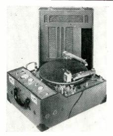
which are modifications of the famous Presto K-8 and Y-2 types. The new units will do standard recording as well as Microgroove, and modifications include an advance ball on the cutting heads and dual purpose pickups. The quality of recording is excellent. The K-8 will record continuously for one-half hour on one side of a 134/4" disc. Microgroove units are offered at no price increase over former types.
