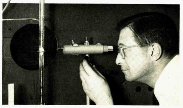
Metallurgist Henry C. Theuerer, M.A. in Chemistry, Columbia, watches a molten zone in a silicon rod under purification. Mr. Theuerer's most recent achievement was development of water-vapor treatment for removal of boron.
