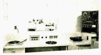
Both changer and transcription turntable play through the amplifier system in this control room. The tape recorder at the right makes it possible to record student activities when desirable.
