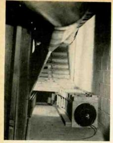
Fig. 2. The throat end of the horn, showing the 15-in. driver.
