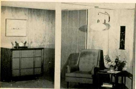
Fig. 3. Interior of listening room, showing mouth of horn. Grille discourages walking into the horn.
