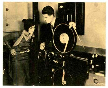
Douglas Shearer shows his sister, actress Norma Shearer, how the voice is photographed on film as it comes through the recording channels in the form of electrical impulses. (*Photo—Courtesy of Western Electric.*)
