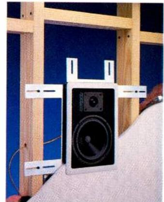
After the walls are installed and finished, the speaker frame is securely attached with the six mounting screws supplied.
