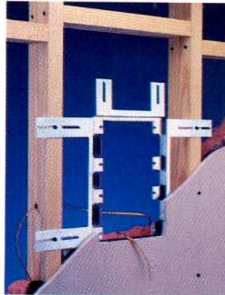
This optional bracket mounts directly to the wall studs, much like an electrical box.
