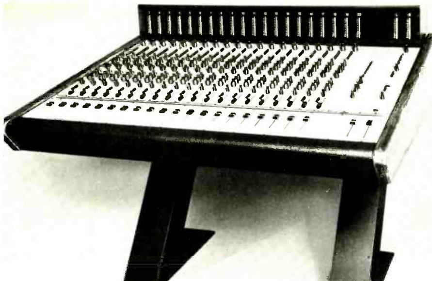
concept and totally modular in construction. The standard main frame has a maximum capacity of 20 in/output modules and is complete with all the necessary master and monitor functions required by the latest multitrack recording techniques.
