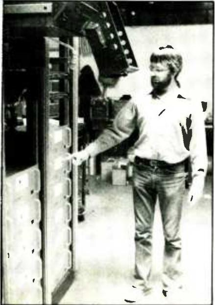
McCune for permanent installation at the Crystal Cathedral includes several features designed to prolong the life of the system, and ensure a minimum of inconvenience when something does go wrong. Magnetic circuit breakers — one for each amplifier, Meyer processor, power supply and blower, and even one for the utility outlet on the front panel — respond much more quickly than the standard variety.
