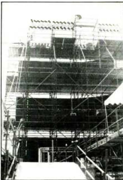
Figure 1: Clair house system comprised 180 S-4 cabinets and 32 long-throw constant-coverage long-throw horns; S-4s were stacked 10 wide and three high on three tiers per side.
