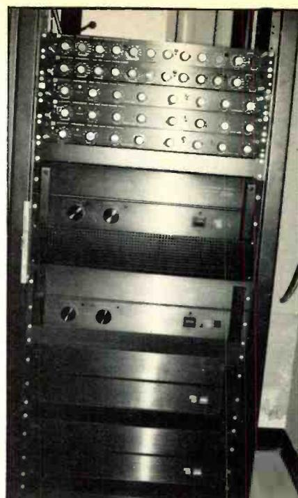
Sound equipment racks house Klark-Technik DN27 third-octave graphics, Technics cassette deck, Sony PCM-F1 processor and U-Matic VCR (left), and a bank of Audio Arts crossovers and AB Systems power amplifiers.
