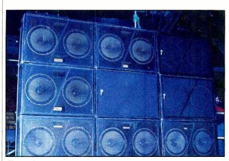
Photo 13. Large-scale concert use requires speaker system components that can fill huge performance spaces. Shown here, Meyer Sound Laboratories' 650-R2 subwoofers as fielded by Ultra-Sound at Meadowlands Arena in New Jersey.
