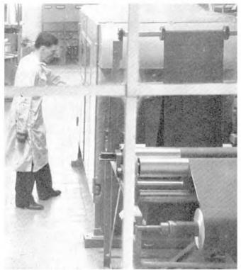
Fig. 3—The film leaves the coating machine in a wide strip.
