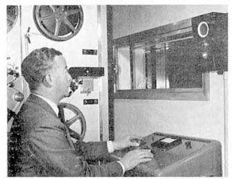
From his control panel the recording engineer can look into the commentary room. The picture is being projected from the panel nearest the window. On the adjoining panel the commentary is being recorded on 16 mm fully coated film. Both these panels are so coupled that it is impossible to lose sync. even when run rapidly in reverse. This makes it simple to re-record a single phrase if the commentator makes a mistake.
