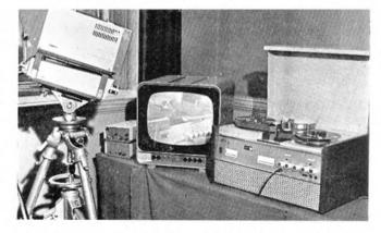
Coupled to its pre-amplifier by a rotating transformer, the head scans 1 in. tape moving at 7½ i/s, at approximately 23 yards per second. Maximum playing time, using 1,800ft. of LP tape, is 45 minutes.
