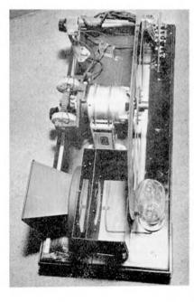
Fig. 5 (left): Televisor mlnus cabinet. Relationship viewing lens, Nipkow disc and lamp can be seen in the foreground.
