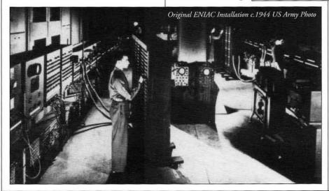
the active circuits were equipped with neon lamps to show the current state and results, although reading these lamps was a job for an experienced operator. Press relations were considered a major part of the project, and so a special lamp panel was built to display the contents of an accumulator for newsreel film crews.
