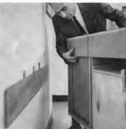
Left: Author Mike Kay is ready to "float" Cabinet on beveled board. Note shims behind board to compensate for uneven wall.
