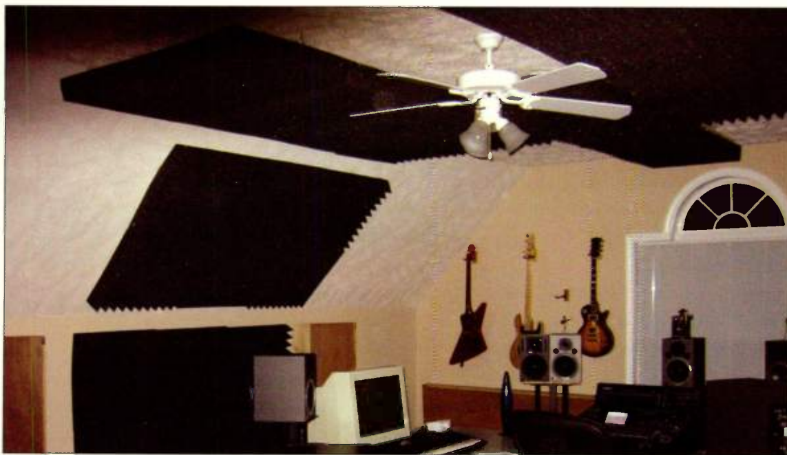
Here we see the finished room, with acoustic panels and bass traps hanging from the side wall, and suspended acoustic panels hanging from the angled side walls and the ceiling. The shape of the cloud has been changed from John Storyk's original rectangular design to allow for the ceiling fan/light fixture and two heating/cooling vents that are in the ceiling near the front of the room.
