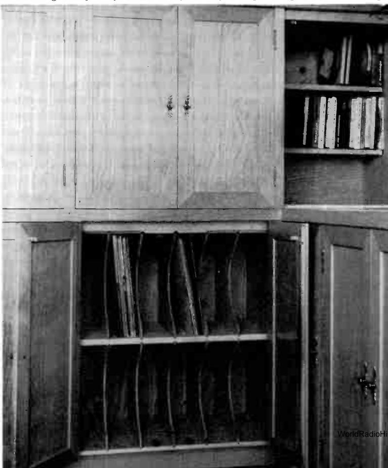
secure the cabinets to the walls with bolts at the rear threaded into expansion plugs. This was done not only to hold the cabinets in place, but to eliminate any cabinet resonance effects or vibration.
