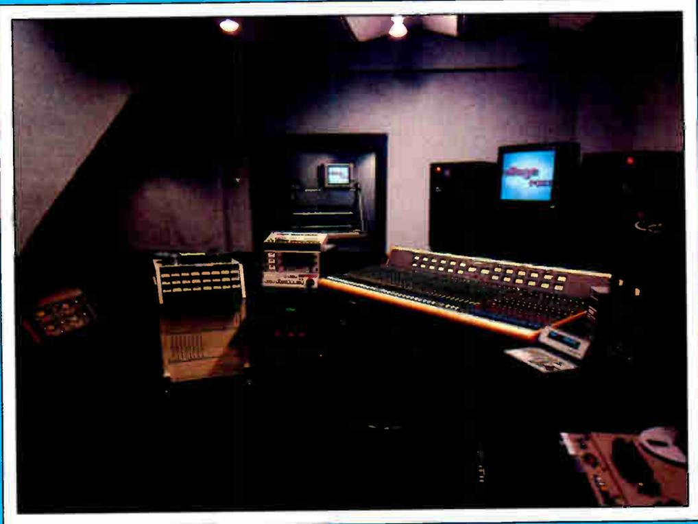
The Village Recorder serves the video post-production needs of its L.A. clients in Studio "F". Shown here are the Trident Series 65 console, an Otari MX80 24-track recorder, 13-inch and 20-inch Sony video monitors and a pair of JBL 4425 monitor speakers. Other equipment includes three TimeLine Lynx synchronizers, a TimeLine Lynx controller and an array of signal processing equipment. Photo: Betsy Annas
