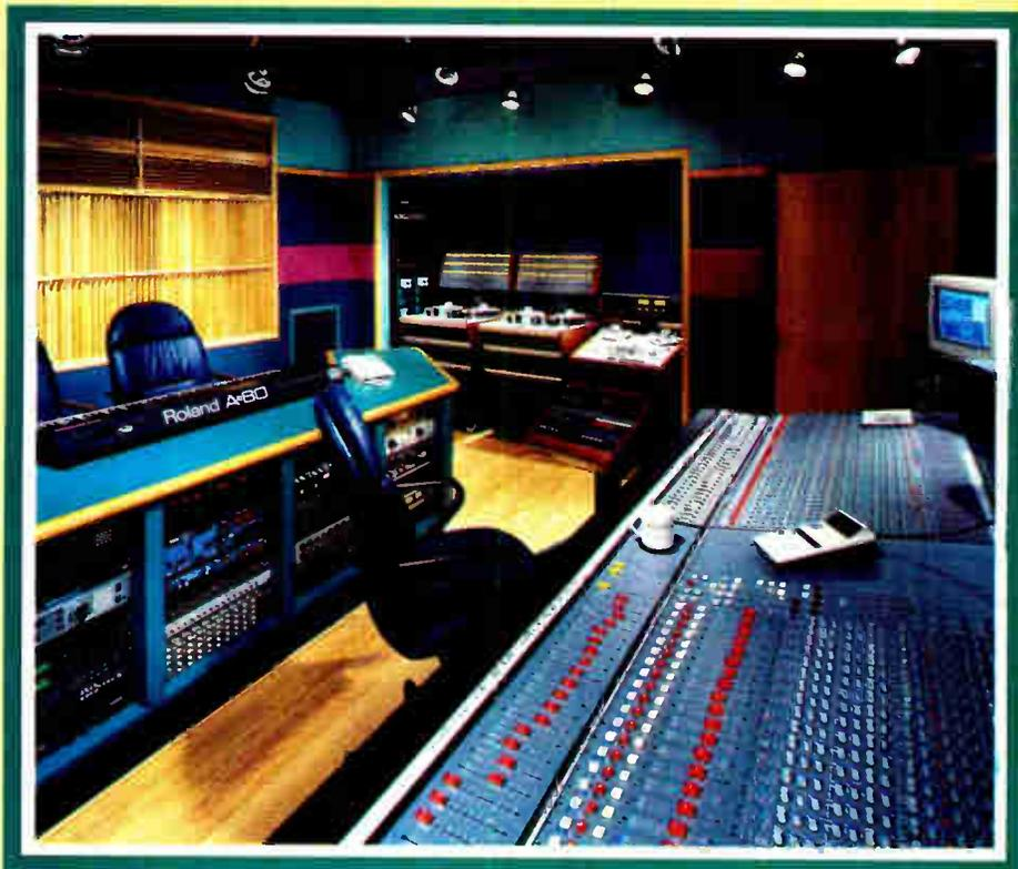
Located outside of Portland in Wilsonville, Ore., Musicon was designed by Russ Berger to function primarily as a music recording room, although it also includes video lockup capabilities. The control room features a DDA AMR24 expanded frame console with bar graph meters on inputs, Studer A827 multitracks and custom diffusers. The main monitor system uses Tannoy System 215 DMT speakers with programable EQ setup by George Augsburger. **Photo:** Galbraith & Wilson.
