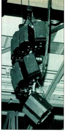
A loudspeaker cluster constructed with ATM flyware.
