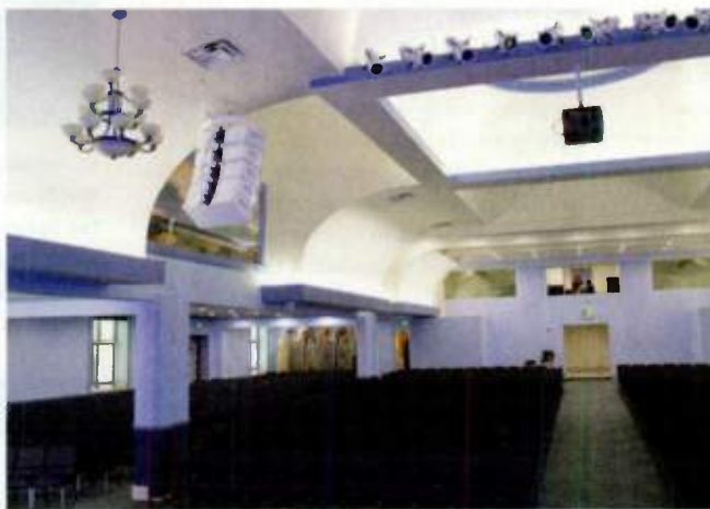
Hanging locations for the VUE Audiotechnik al-8 arrays were limited by the architectural features at World Agape Mission Church in Los Angeles, where VUE a-8w speakers provide coverage for the side seating area, which has a 9-foot ceiling.
