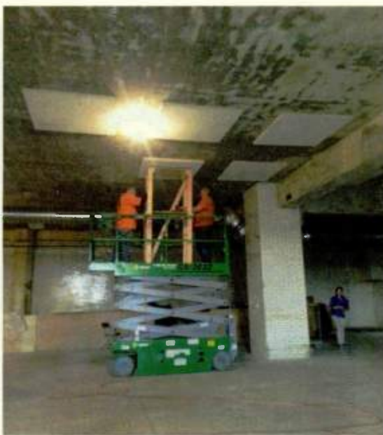
Pearl Pro Audio installed dozens of Tectum Finale sound absorption panels inside the Old Bakery Beer Brewery in Alton, IL
