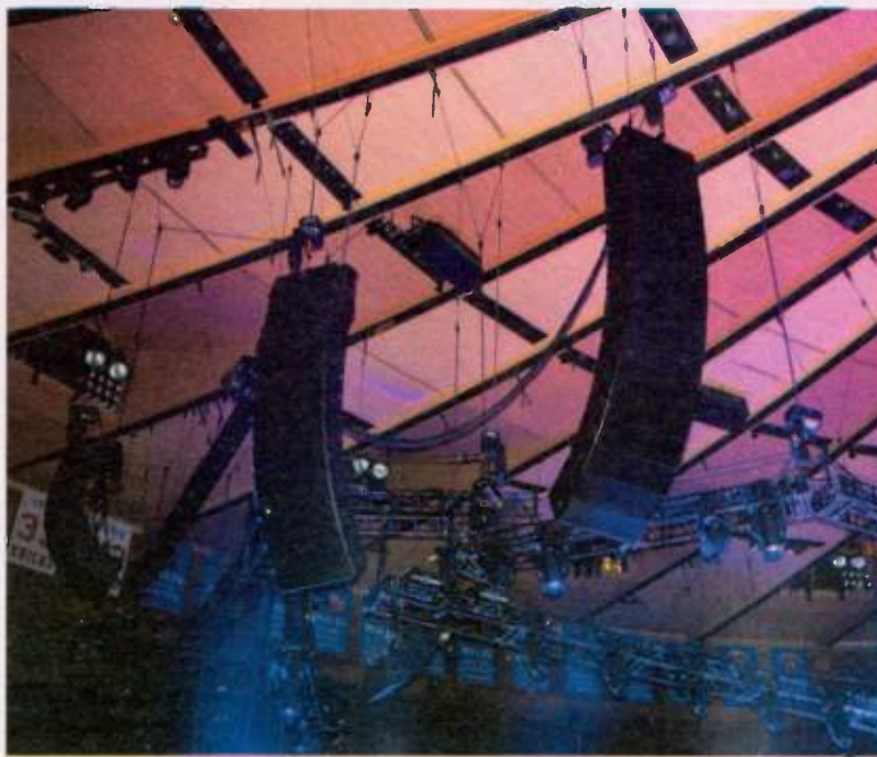
A d&b audiotechnik P.A. based on the flagship GSL System (right) and both J and V Series boxes for side hangs.
