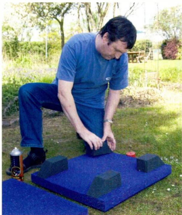
Normally acoustic foam panels will act primarily on mid-range and high-frequency reflections, but you can improve the low-frequency absorption effects by spacing the panels a few inches from the wall surface — the easiest way to do this is simply to stick small off-cuts of foam to the back of each panel as spacers (left). For best results, fix the panels across the room's corners (right).
